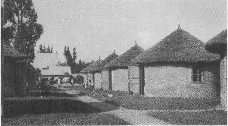
Figure 2. Tukules in "the Children Street Section" of the hospital built by the Italians.
